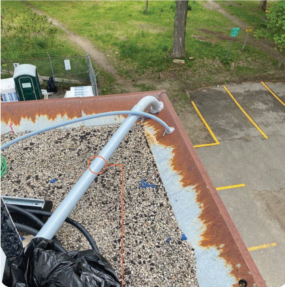
Wiring Set Up To The Building
