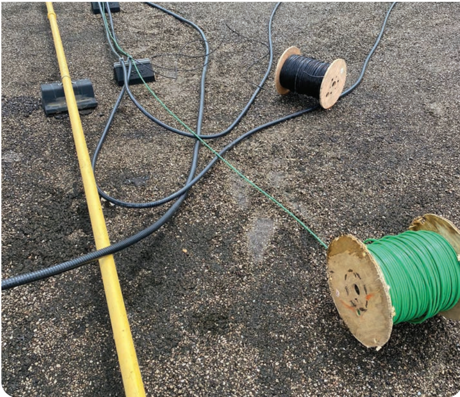
Wiring run to the electrical room.
