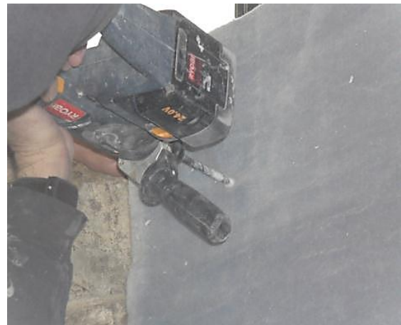
Drilling Spaceloft® - 40mm layer
