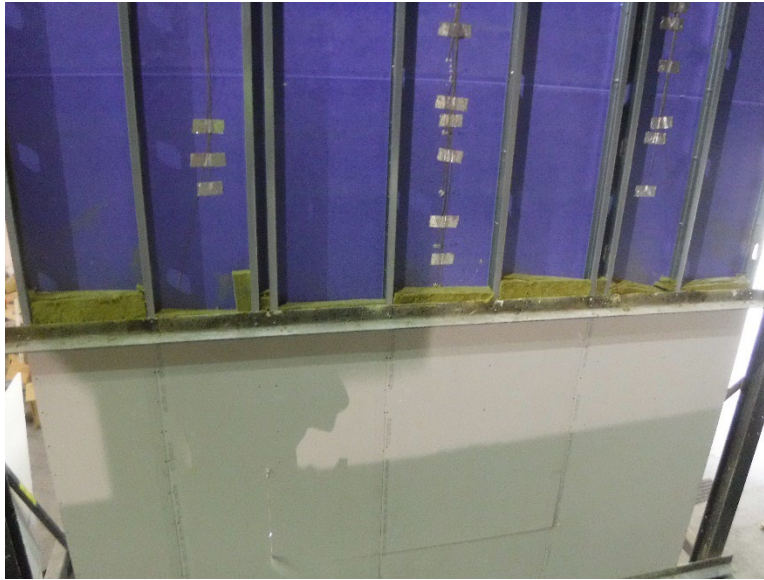
Photo No. 5 Floor Safing Installation
