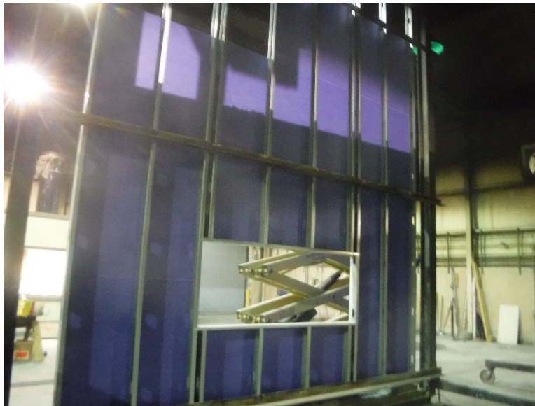
Photo No. 1 Core Wall Construction
