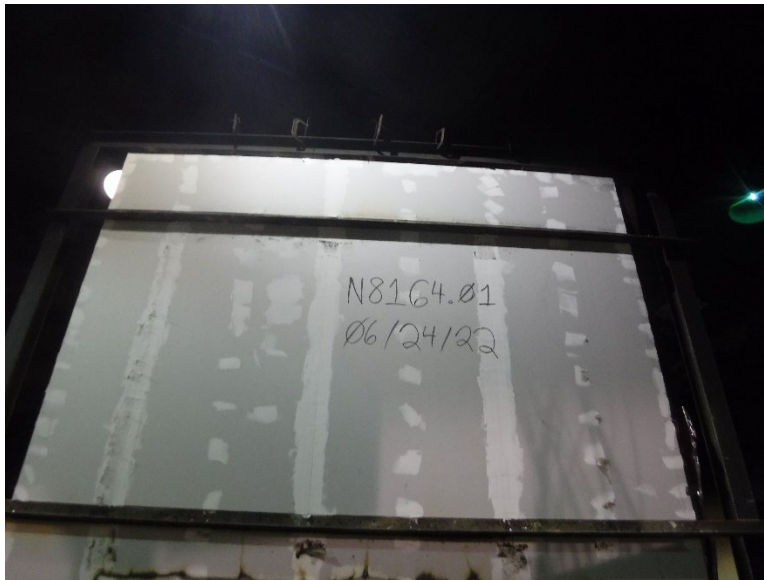
Photo No. 19 Second Story Interior Gypsum (Post-Test)
