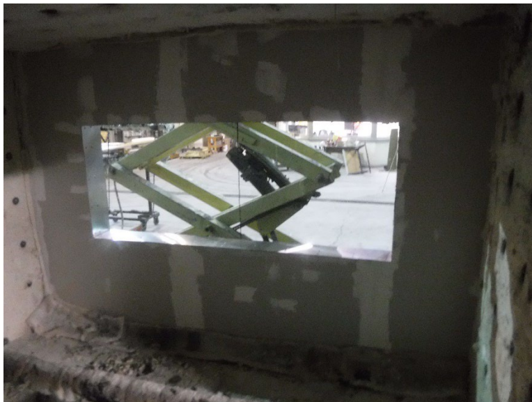
Photo No. 8 First Story Interior Gypsum (Pre-Test)
