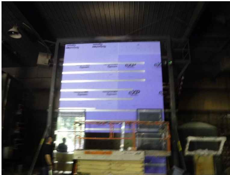
Photo No. 3 Installation of the Horizontal Rails
