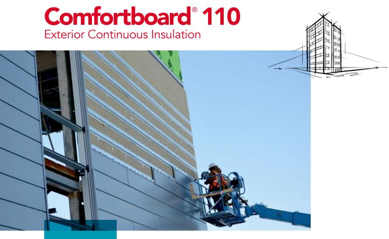
ROCKWOOL Comfortboard® 110 is a rigid, high-density, non-combustible stone wool insulation board designed for use as an exterior continuous insulation in commercial applications.
