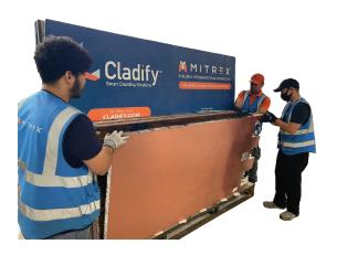
8. One by one, lift each remaining module and place it in a dry and safe place until it's installation. Do the same for the remaining modules until the A-frame is empty.
