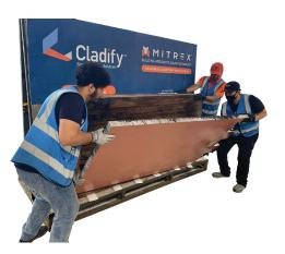
**WARNING:** The glass facing of the module can be damaged if it is not placed properly. Make sure that if the panel is facing down, there is not any screw or metallic piece that can damage the surface.
