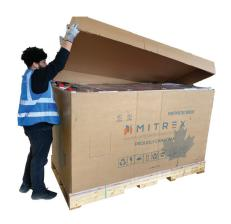
4. With a partners help, remove the box that is covering the panels by lifting it. Put it aside.
