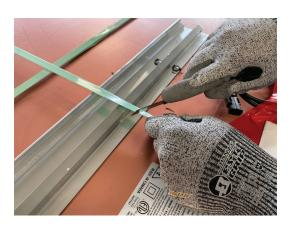
7. Cut the vertical straps (2. and 3.). Make sure you do not cut or damage the honeycomb or glass facing.
