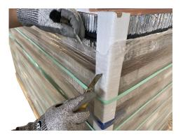
10. Remove the first corner piece by pulling the piece downwards. Only remove the corner pieces covering the top 2 panels. Repeat this in the 4 corners.
