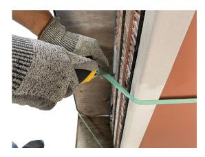
5. Then cut the second strap. Make sure the modules are held by your partner at all times during the cutting to ensure the modules do not fall to the floor.
